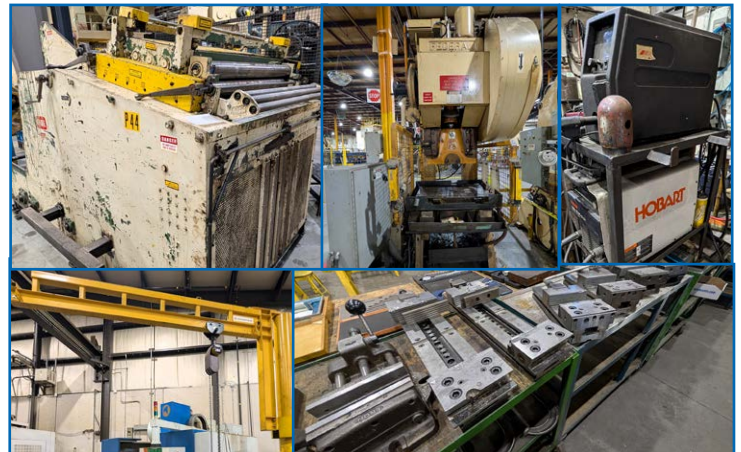
PARTIAL VIEW OF SUPPORT EQUIPMENT
